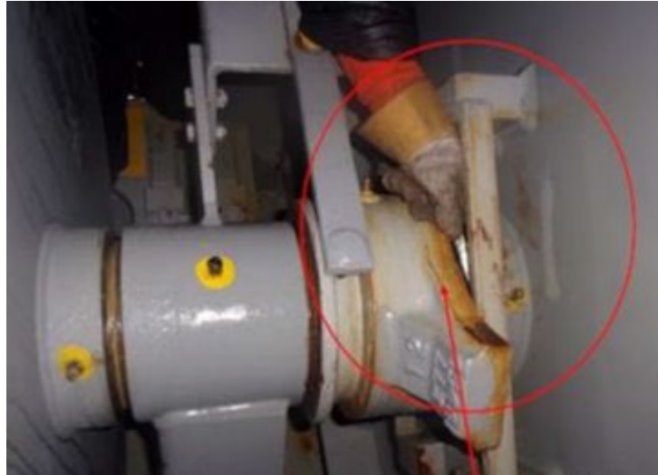
Position of hand during injury. Removing old grease using short length hacksaw blade
