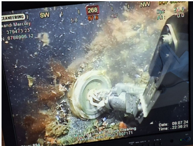
Cleaning of 159mm Dia chain prior installing cutting tool
