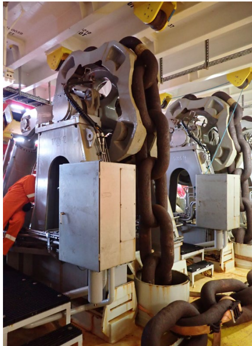
Function testing of mooring winches
