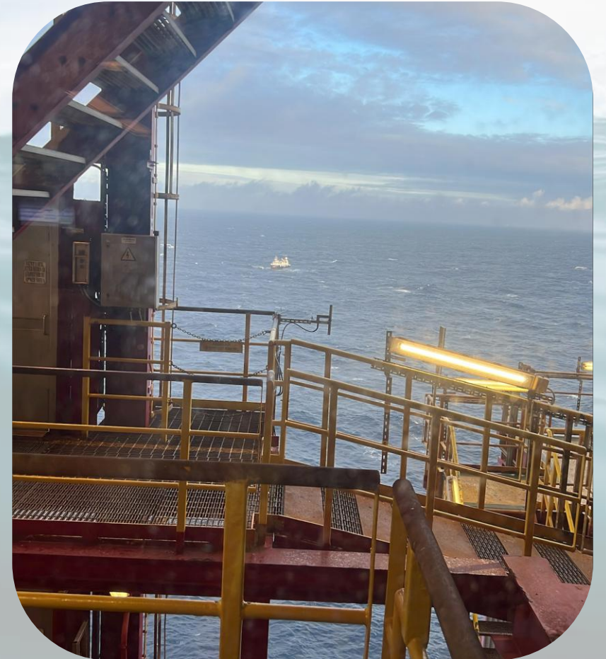
Reach Remote 1 at Gullfaks C, 10.03.26
